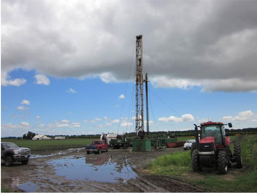
**Photo 5:** Drilling work at the saltwater disposal well site.
