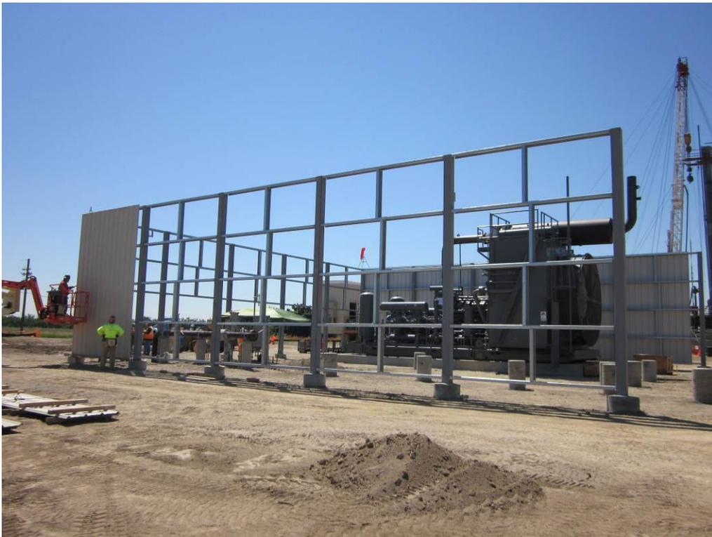
**Photo 2:** Soundwall work at temporary compressor placed at the remote well pad site.
